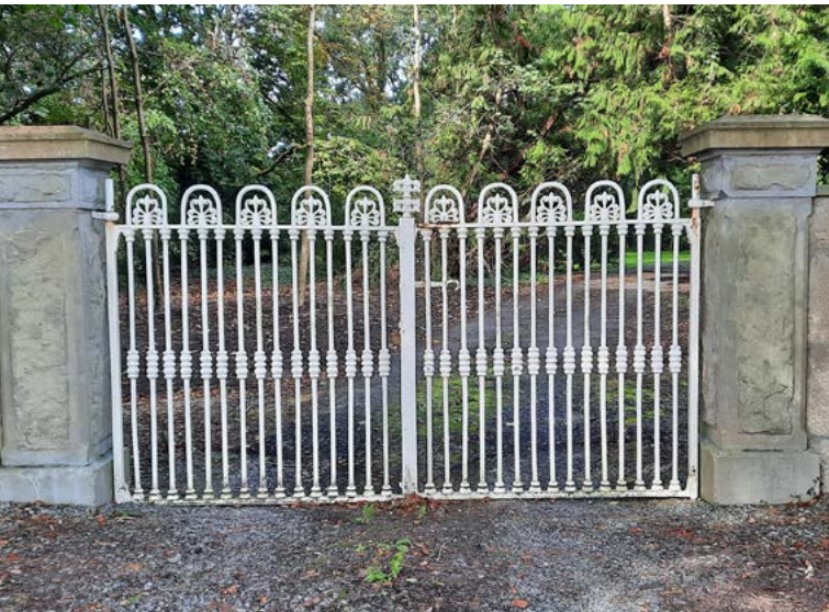
Bell's House forged gates, made by Bannerton Blacksmiths, Ahascragh, County Galway.
