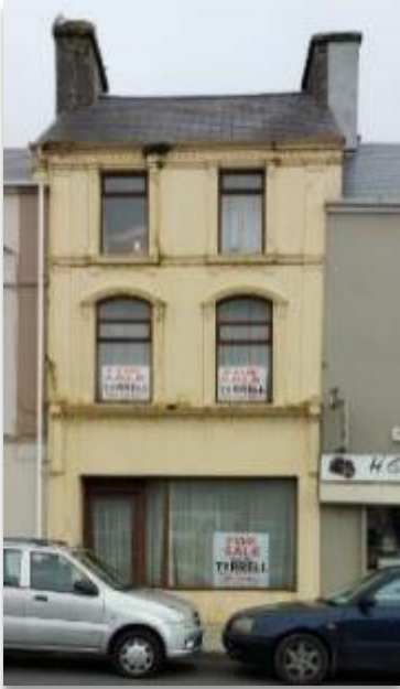
Photograph: An unusually narrow three storey, two bay building with integral shopfront, the Square, Dunmore
