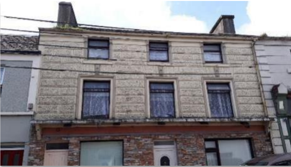
Photograph: Plaster decoration on lined and rendered façade of upper floors of house in Castle St. with remains of fascia of a traditional shopfront over ground floor.
