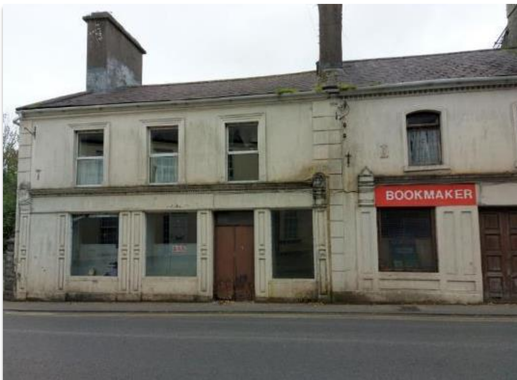
Photograph: Former houses with integral shopfronts, Bridge St., Dunmore
