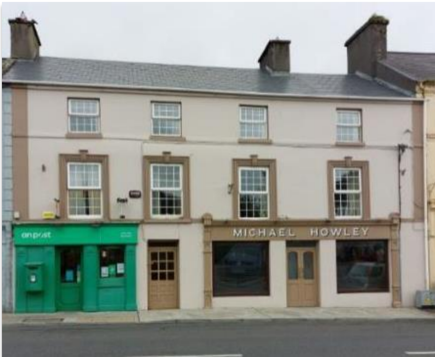
Photograph: Traditional shopfront with hand painted name plate and modern post office shopfront set into ground floor of house. Second floor windows with decorative channelled architrave with central pediment.
